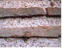
Roman mortar (Trier, Germany). Made of white lime and red powdered brick (testa in Latin). The «testa» contains the elements necessary to start the geopolymeric reaction and the hardening of the mortar.
