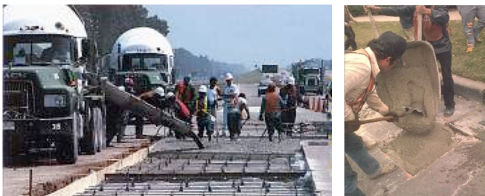
Figure 11!: Use of PYRAMENT in USA as pavement repair material
