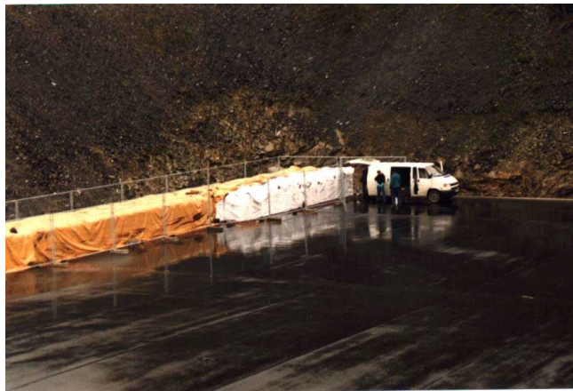
Big Bags with Geopolymer® blocks on prepared landfill
